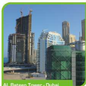
AL Bateen Tower - Dubai
